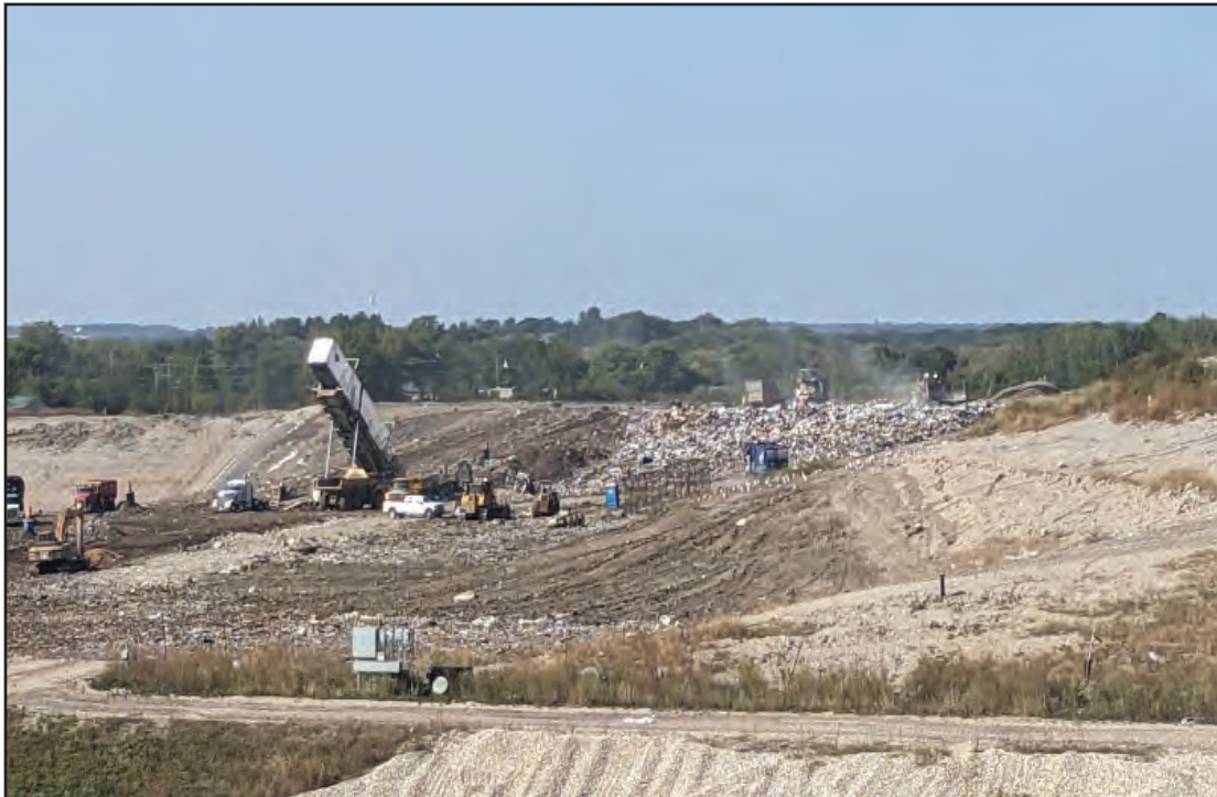
Working face at North end of Phase 3, overlaying on to Phase 2
