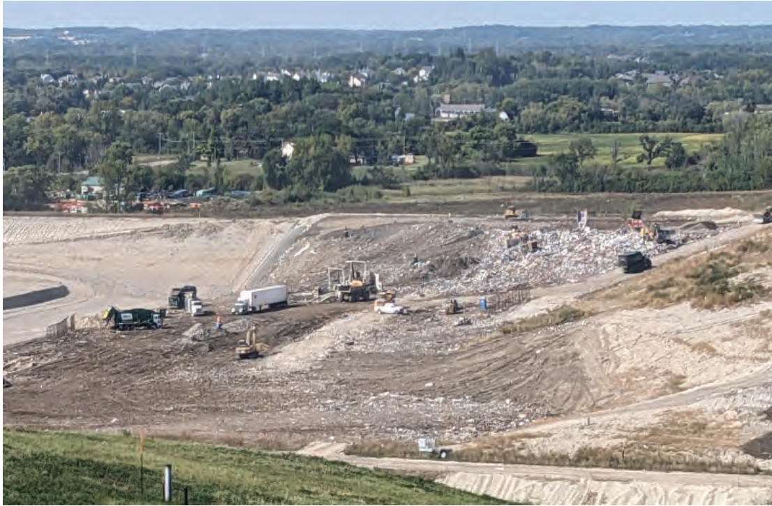
Phase 3 receiving waste
