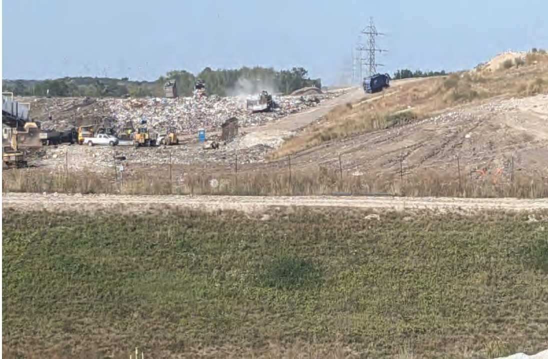
Working face at North end of Phase 3, waste mass nearly cresting
