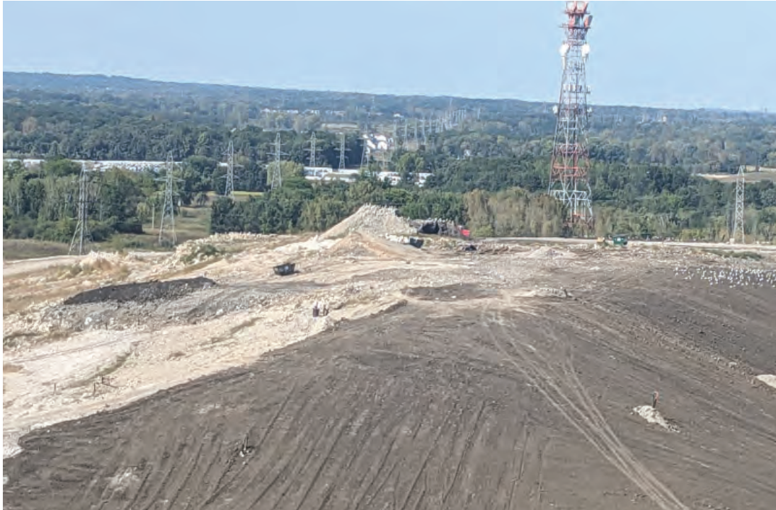
Working face at North end of Phase, being covered
