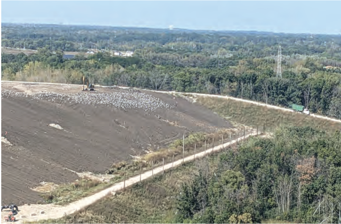
East slope of Phase 1 top soil cover for vegetation growth
