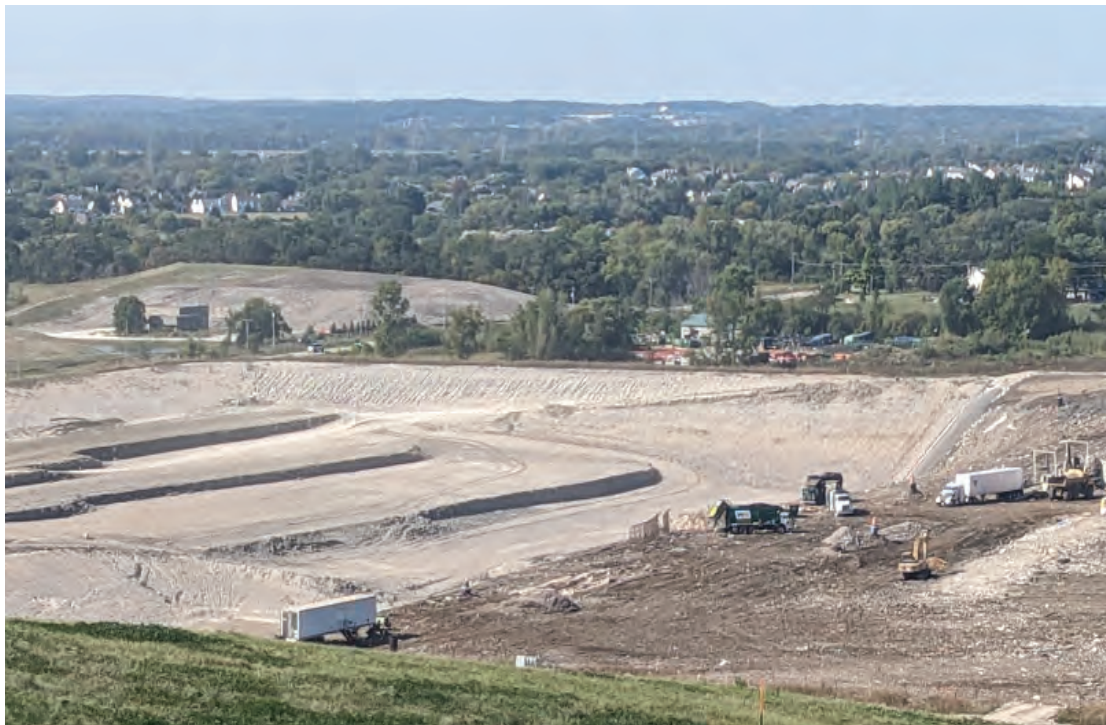
Previous lift across Phase 3 and future cell location
